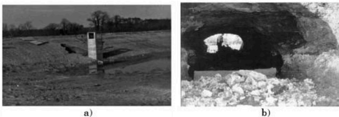
**Figure II.4** – Dam failure caused by concentrated leak erosion (Fell and Fry, 2013)
